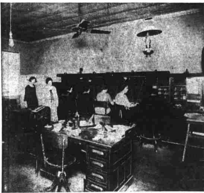
"Number, Please" first sounded over telephone wires in Big Spring from this board. It was the original telephone exchange of the city, installed early in the 20th century when C. E. Alderman, who died recently in Ohio, organized the Western Telephone company. The exchange was well equipped, providing for five operators in addition to additional staff members. Evidently the telephone company wasn't any surer of the electric service than the public was of the telephone service for while an electric light bulb dangled from the drop at the left, a coal oil lamp was ready for emergency service at the right.
