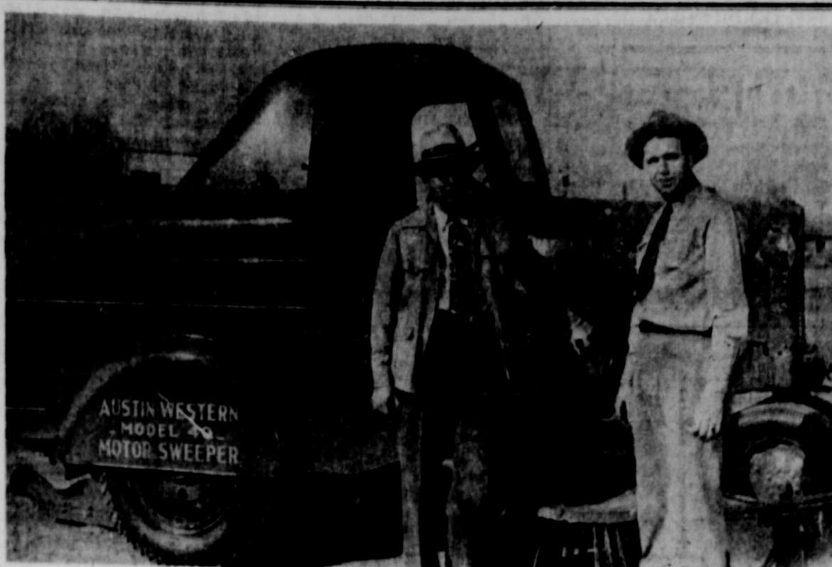
PERRYTON'S STREET SWEEPER—This is the machine that is expected to keep dirt and debris off Perryton streets. It is the new $7,240 Austin Western motor sweeper, the latest thing in dirt removing. Shown by the machine are E. L. Mitchell of Lubbock, company sales representative, and Mayor Rufus Bolerjack. The machine has a hopper which holds two cubic yards of dirt and is designed to sweep close to curbs.
