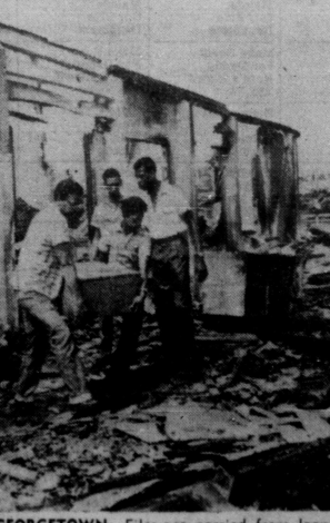
CLEANING UP IN GEORGETOWN—Files are carried from loan association office in Georgetown, British Guiana. Building was among those destroyed by huge fires in heart of city during recent anti-government riots. British troops were flown to the colonial capital to restore order. (AP Wirephoto).
