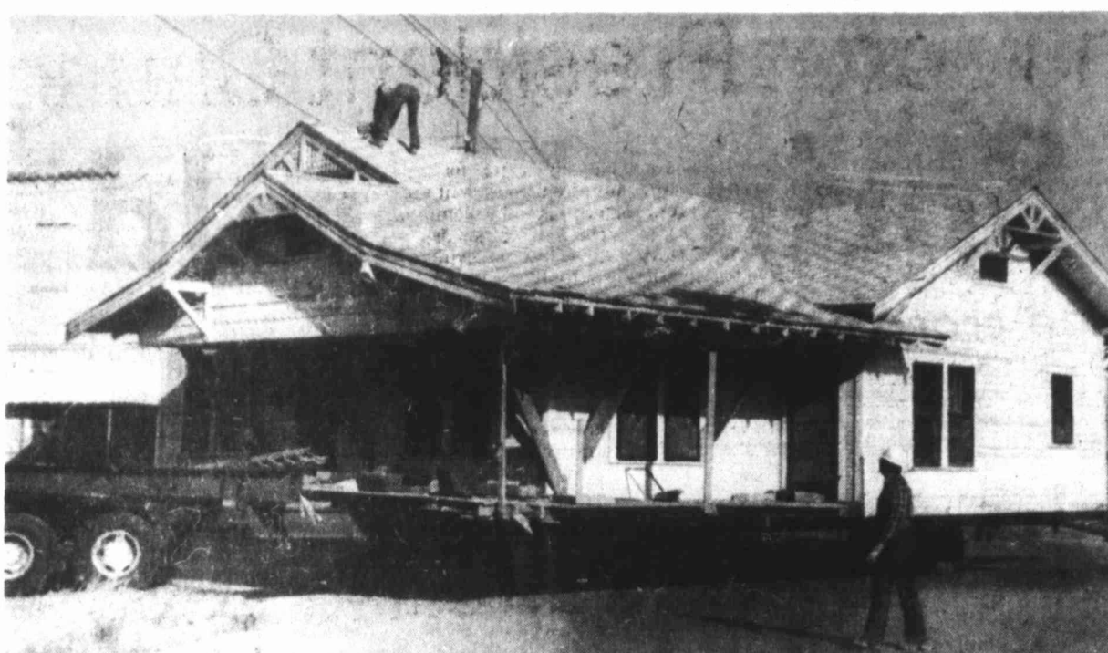
LANDMARK REMOVED — Movers were busy this morning removing the house once occupied by the late Mr. and Mrs. Sam Hathcock at 611 Scurry Street. The structure was purchased by James Baker of Coahoma from J and B Investments, a development and law firm owned by Bob Moore and John Burgess. Moore and Burgess have acquired 200 frontal feet or four lots in the block, which they intend to develop as commercial property.
