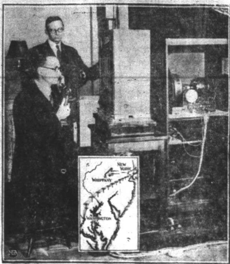
Here is the transmitting apparatus of television. "Electric eyes" are mounted in the cabinet before which R. C. Mathies is sitting. To the right is mechanism which electrifies the image these "eyes" see. Inset is a diagram of the Washington to New York television hookup. Either telephone wires or the Whippany, N. J., radio plant are used for transmission.
