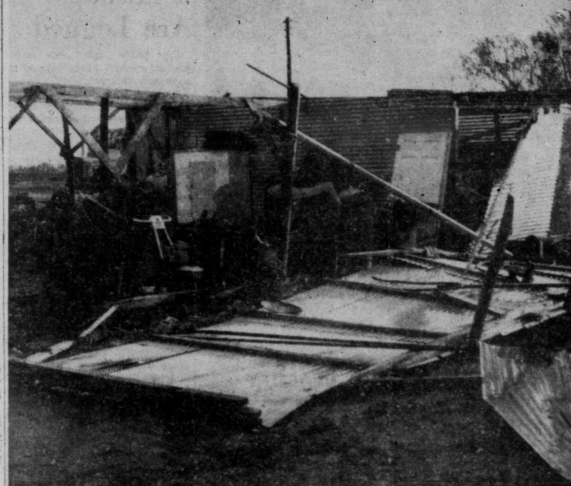
HIGH WINDS LEAVE MARK —High winds produced by a thunderstorm here Sunday afternoon wrecked this building at the J. W. Voss residence on the Big Spring Highway. Several other buildings in Snyder were damaged by the winds which were accompanied by rain and hail.
