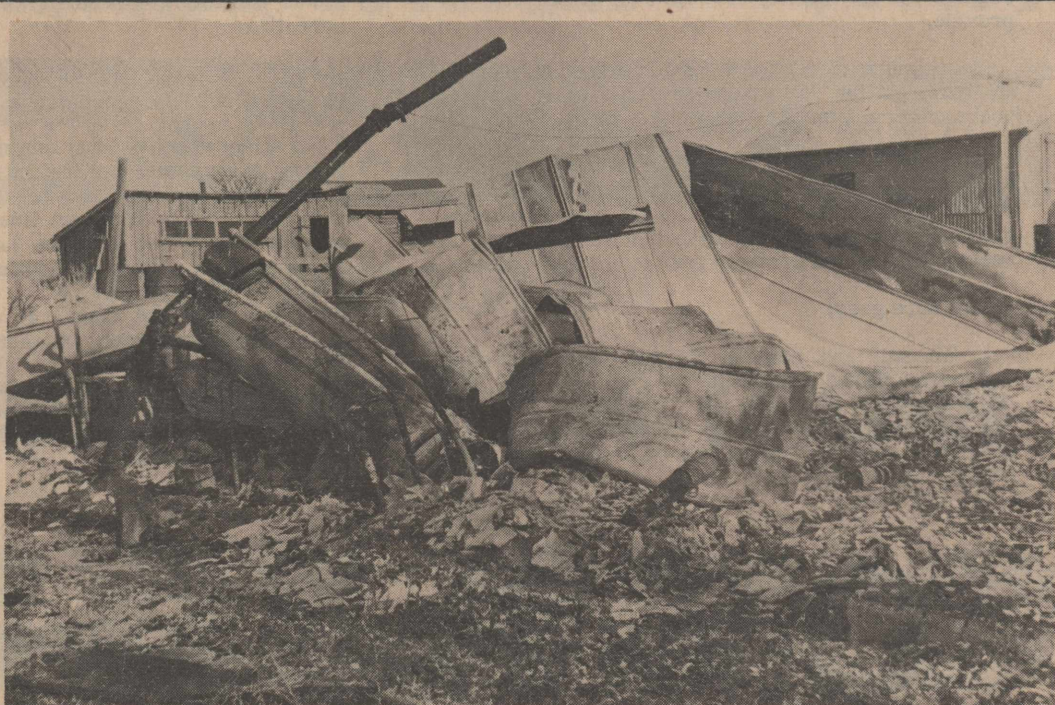
REMAINS OF HOUSE—This was all that remained of a rent house on the E. E. Givens farm, one and one-half miles west of Olton, after a Friday fire swept through the building. The fire was one of three that caused heavy damage over the New Year holiday.
