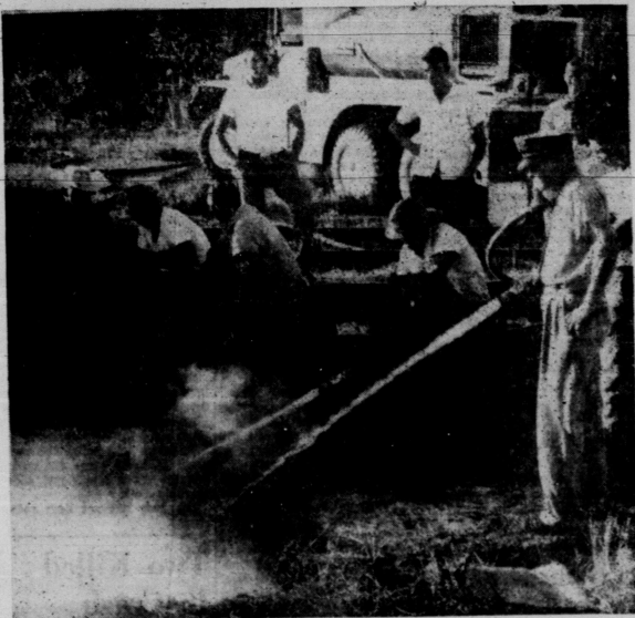
AFTER THE SPACE under the bridge was sealed off, Snyder firemen opened a hole in the top of the bridge, and are shown here flooding the space under the bridge, thus drowning the fire. This technique of fire-fighting is seldom possible, and is probably never taught at fire-fighting schools, but proved most effective in this case.
