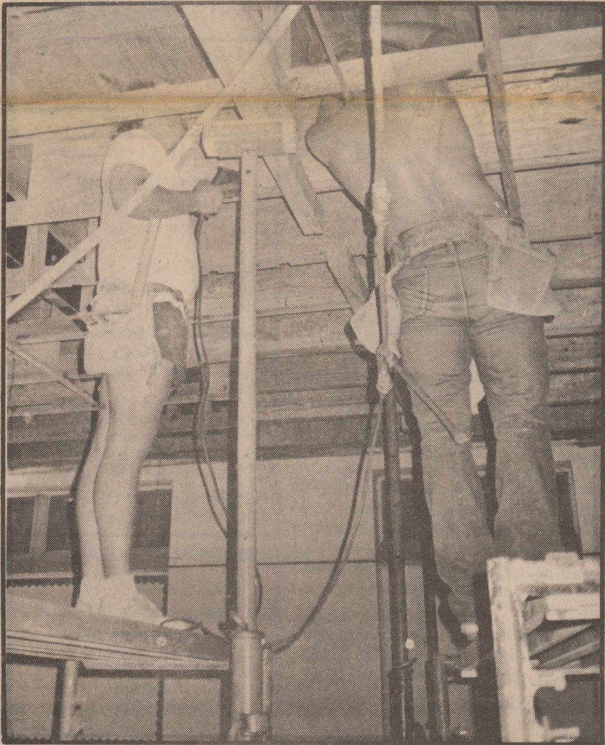
SCHOOL BUILDING REPAIRS: Above are two workers making final repairs on the Rotan Elementary building. All repairs are to be finished by Friday.
