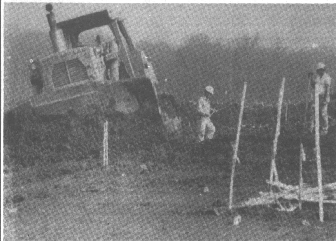
Workmen using earth-moving equipment check the day's progress earlier this week as the clear the site for the Saturn automobile plant near Spring Hill in middle Tennessee. (AP Laserphoto)
