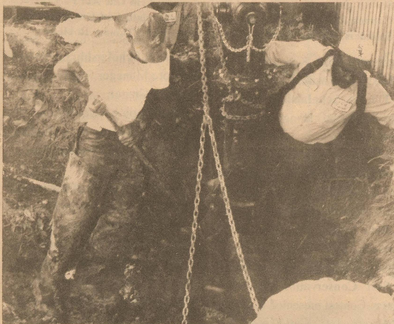
City crews work diligently to repair broken water main near the Woolen Mill.
