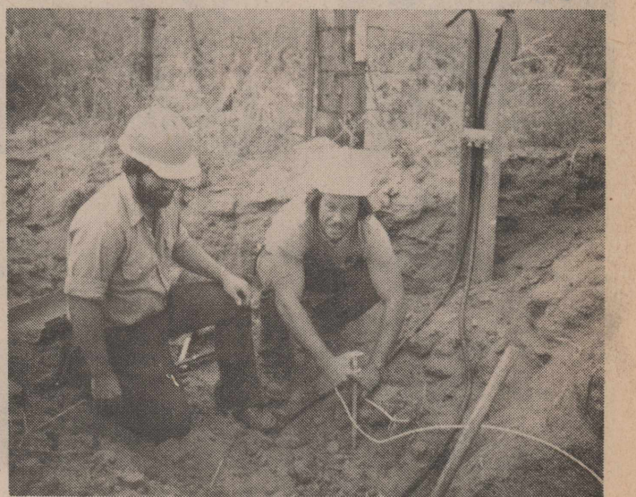
MEN LAYING TELEPHONE CABLE
