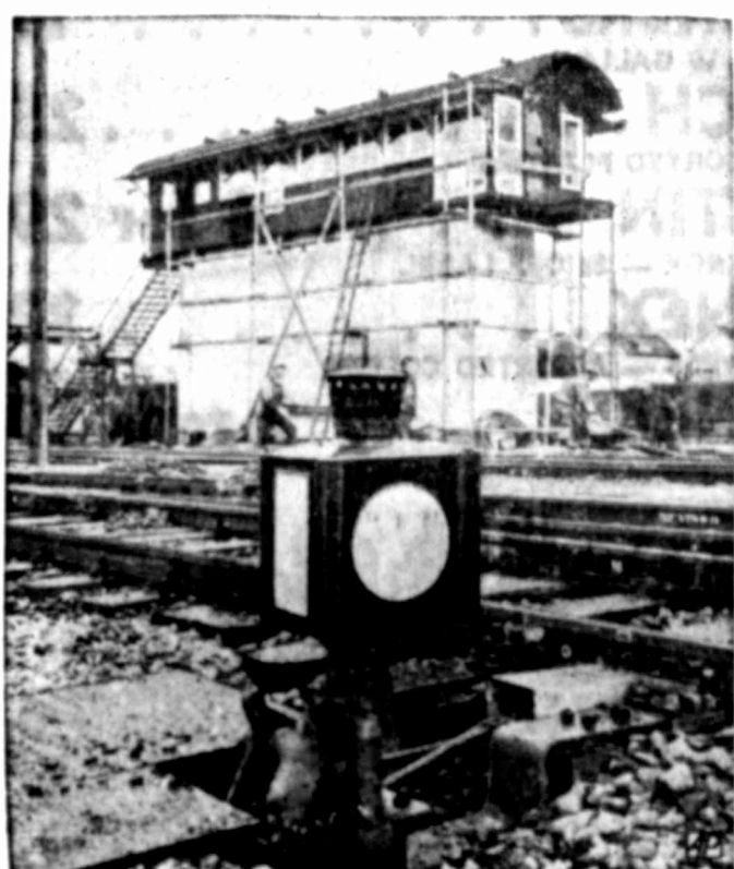
SAVING STOCK —An old railway carriage, after installation of technical equipment, now serves as a rail signal box along track in Stuttgart, West Germany.
