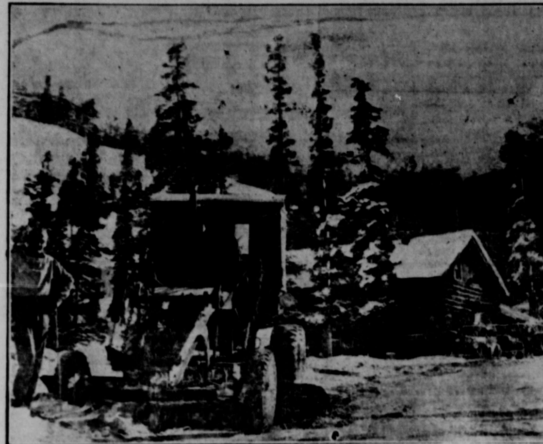
Keeping the world's highest automobile highway open up Pike's Peak is done by modern machinery. Development of the nation's newest winter playground on Pike's Peak gave the fiscal service the snow clearing job. In the background is one of the lodge buildings at the Broadmoor-Glen Echo courses, less than an hour from the mild-weather golfing in Colorado Springs, Colo., and fashionable Broadmoor. Count Philippe de Fret, European skier, is standing beside the snow plow.
