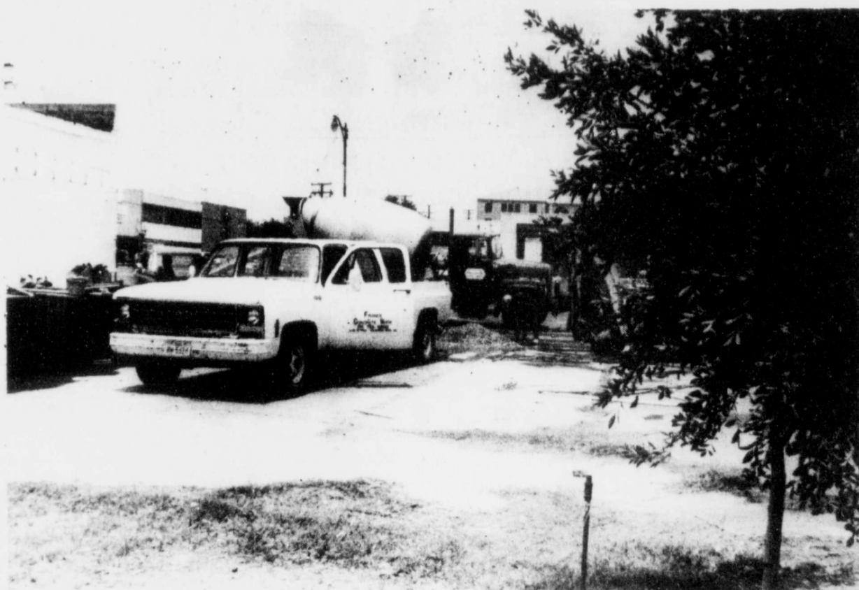
FRANCO & FRANCO have contracted to do the concrete work at the Dell Barber park and gazebo and are setting forms for the sidewalk. Water lines have already been laid and the park is nearing completion.
