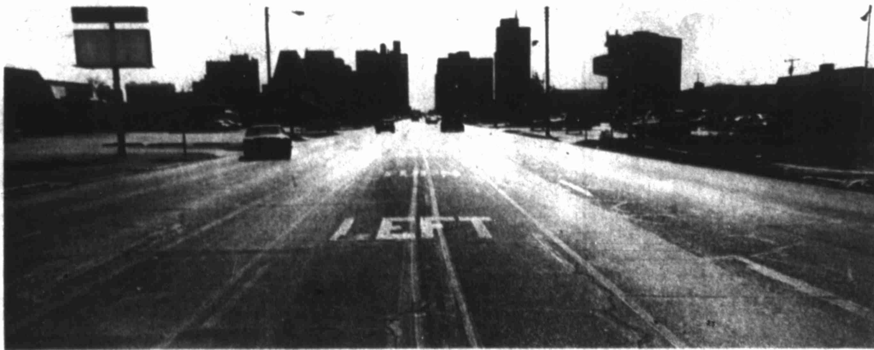
This section of North Big Spring Street near Kansas Avenue not only has badly worn stripes, but a confusing double center line.
