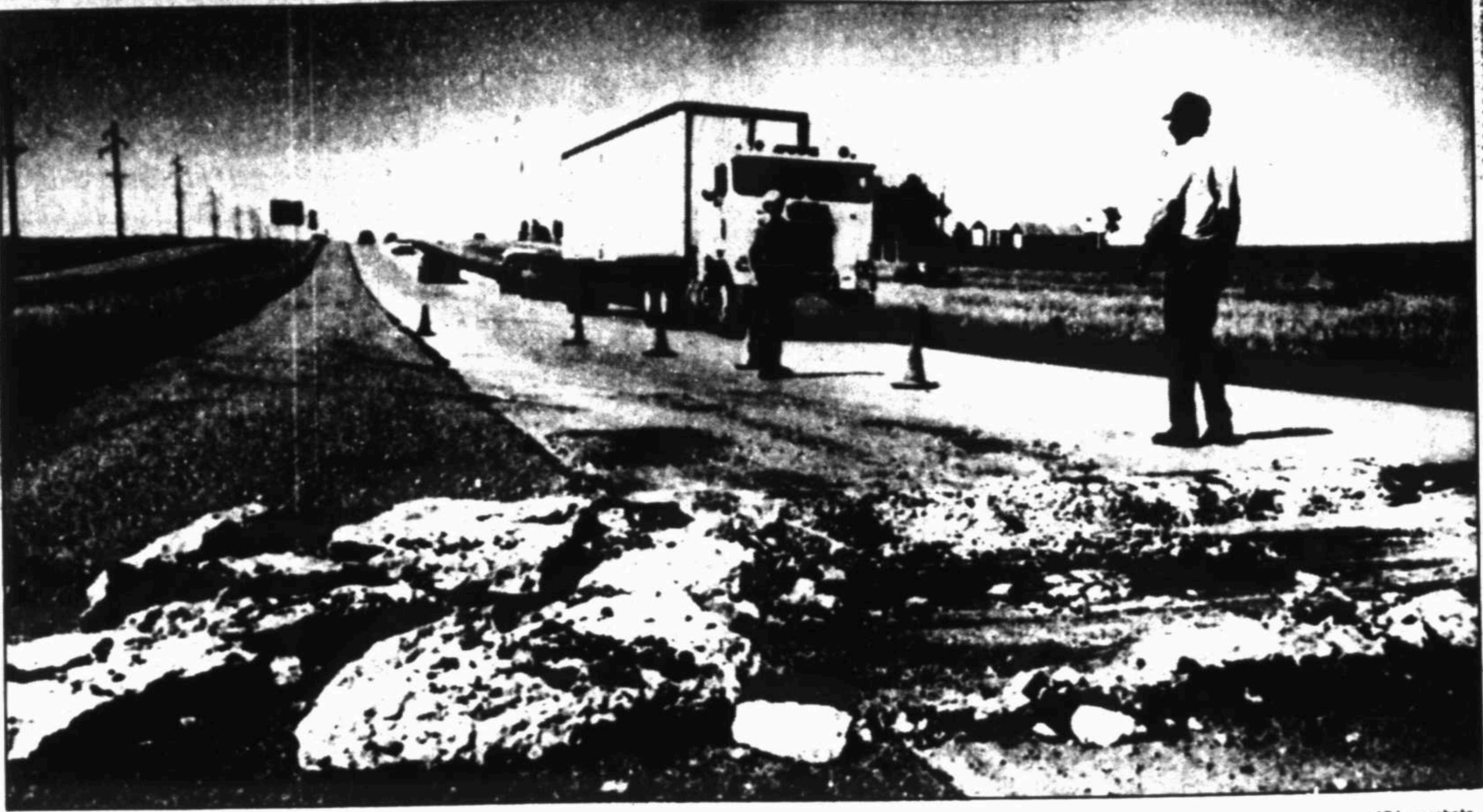
Workers from the South Dakota Division of Highways direct cars and trucks around a portion of Interstate Highway 90 that broke apart in Wednesday's heat. Hot weather caused the cement to expand and crack — a common problem, according to highway engineers.
