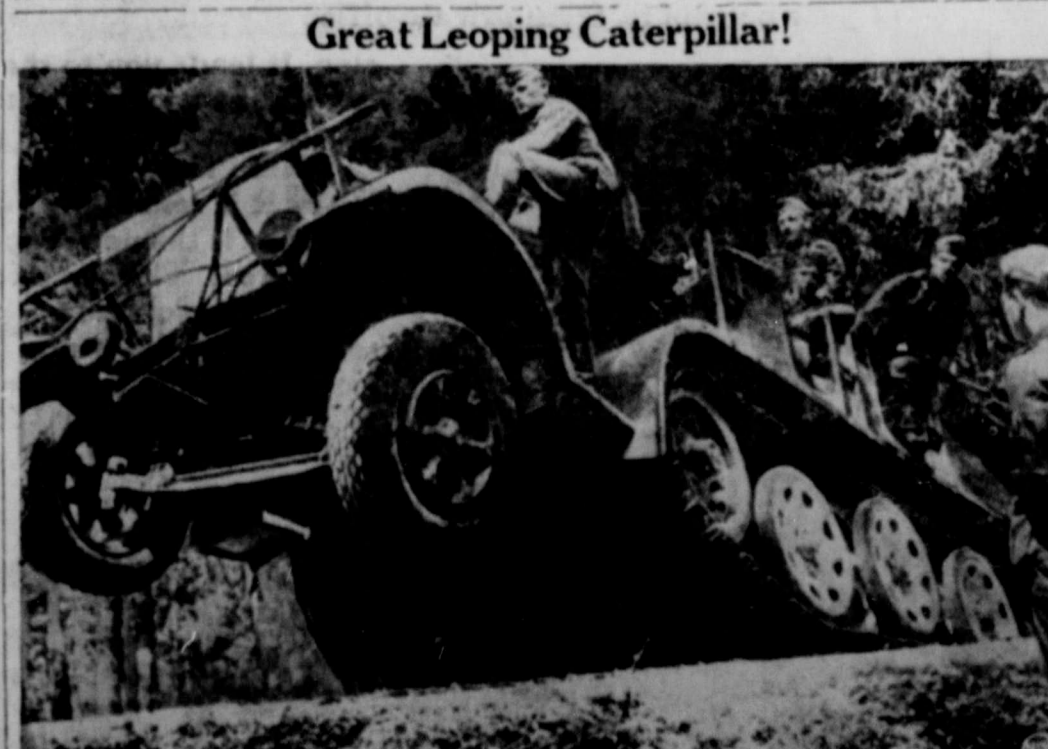
German censor-approved picture shows new caterpillar troop transport with front part apparently capable of being hoisted to make the going easier in winter-time Russia. Part with caterpillar tread then supplies traction, power and direction.
