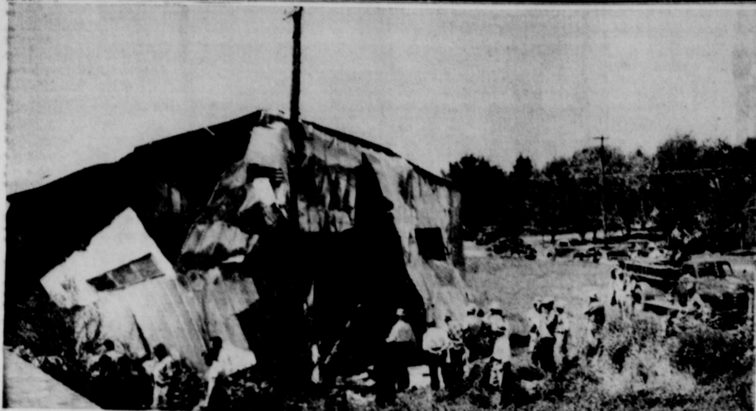
WRECKED BUILDING—Accumulated gas from a broken gas line at the rear of this building was blamed for the explosion which wrecked it Thursday afternoon. The building is owned by the Canadian Truck Line, which recently purchased it from the VFW. None of the truck line equipment had been moved to the building by owner James Pitts. However, much equipment of the VFW post and Auxiliary, which had been left in the building temporarily, was destroyed.
