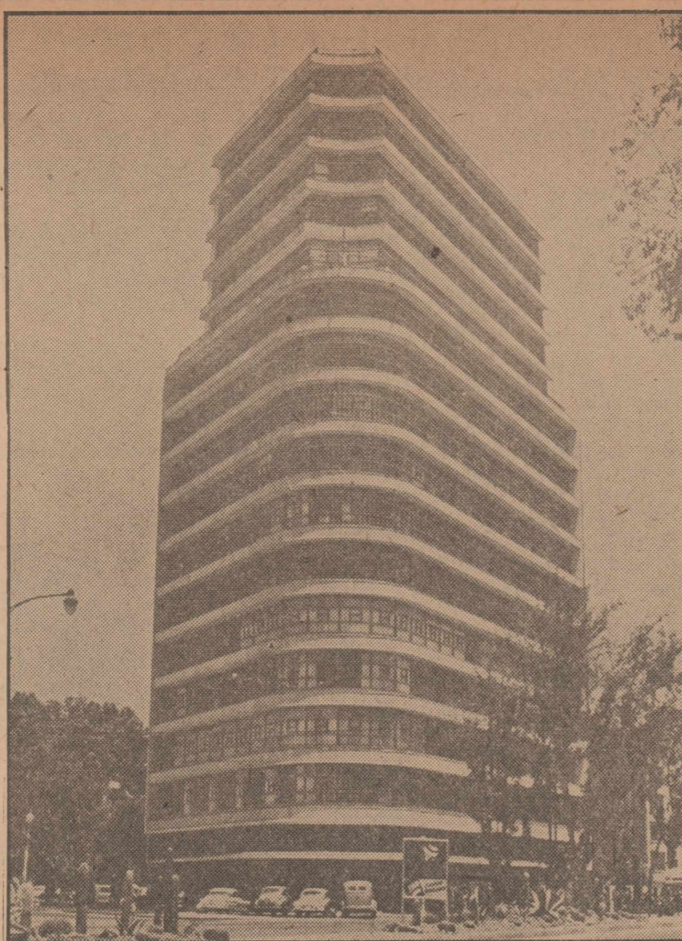
BIGGER AND BETTER —Previously scattered in four different buildings, the U. S. Embassy in Mexico now occupies this modern 17-story structure on the Paseo de la Reforma in Mexico City. The only U. S. Embassy in the world larger than this one is in England.
