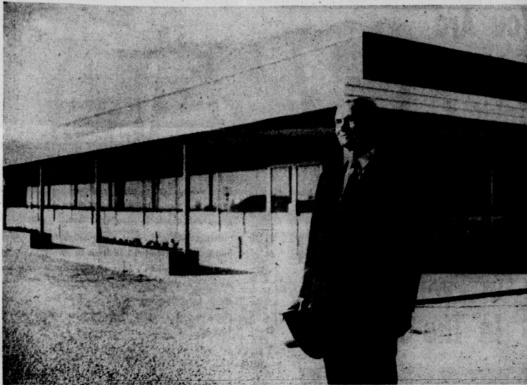
BETTER LIVING, INC., HEADQUARTERS —D. M. Cogdell Sr., who has developed properties in the Cogdell Center area of South Snyder, looks over the new building he has constructed to house Better Living, Inc., a new
