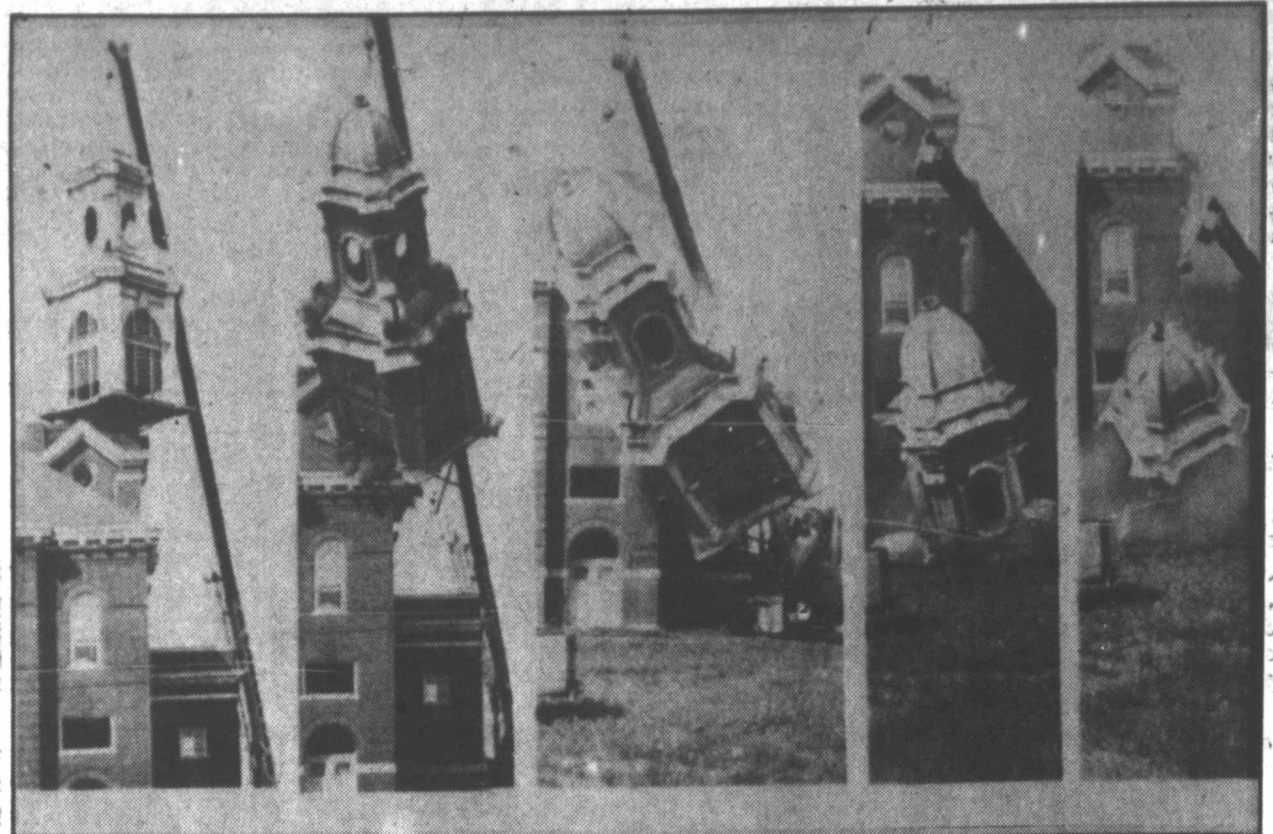
Workmen, using a large crane, attempt to remove the steeple on the former St. Stanislaus Catholic Church in Superior, Wisconsin, in one piece. But the weight of the
