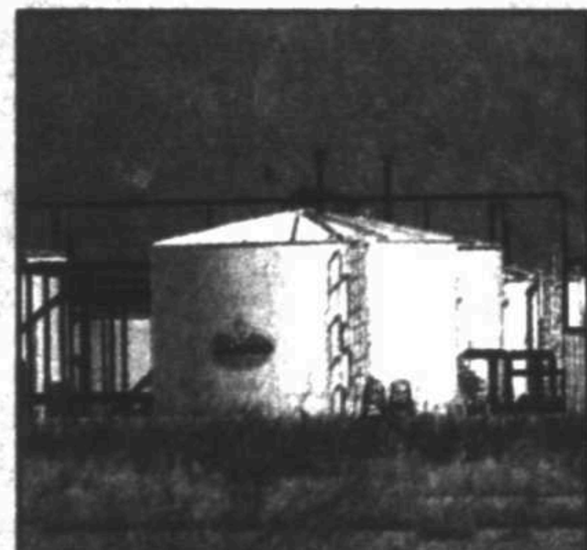
A Tank battery at Amoco's Goldsmith Unit.
