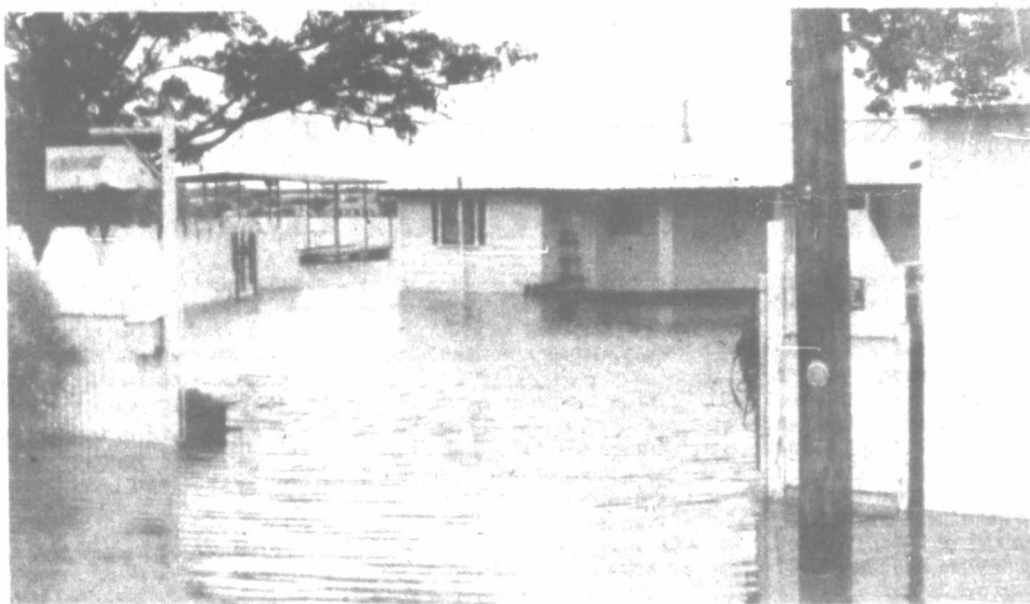
THE LAKE CABIN of A. W. Rowe of Colorado City had water lapping at its back door Monday as the waters of Lake Colorado City continued to rise after recent flooding in the area.
