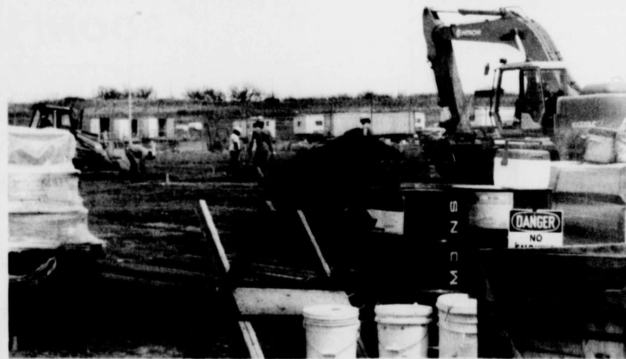
ANOTHER 316 BEDS GOING UP: Turner Construction has begun work on the 316-bed dormitory facility to be built within the confines of the Wallace Unit. The structure will contain 47,000 square feet with 36,000 on the bottom floor and 11,000 on the mezzanine. The inmates confined to these units will share the same dining and laundry facilities but will not co-mingle with the other inmates at the Wallace Unit. This unit will employ approximately 30 additional personnel.
