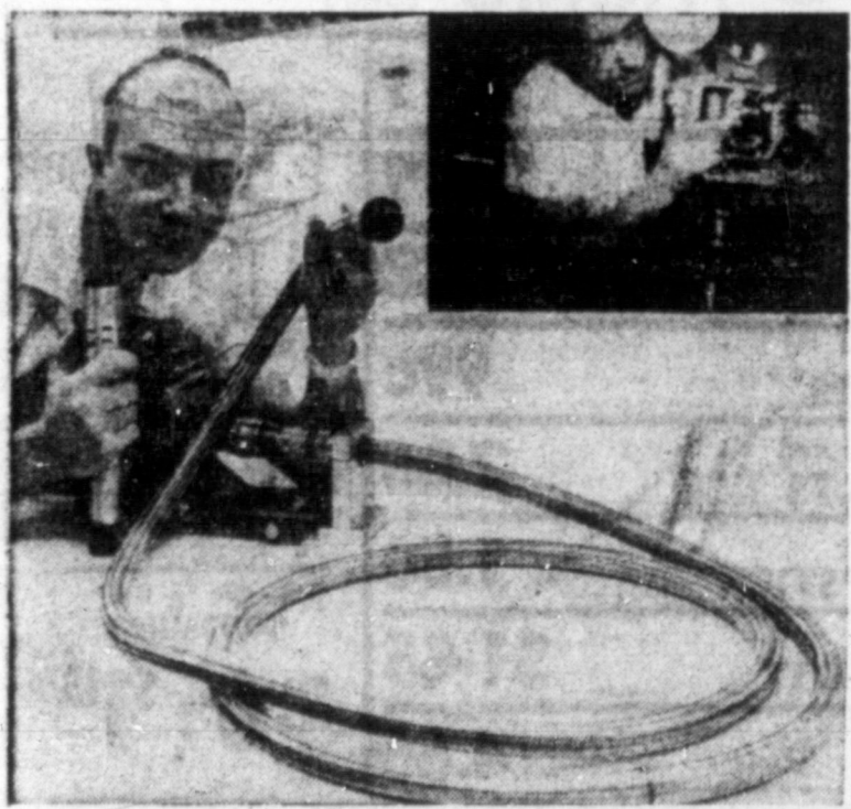
COILED CAMERA—Holding what looks like the end of a garden hose, Milton Rhodes of the NASA Marshall Space Flight Center in Huntsville, Ala., aims a fiber-optics camera at photographer, Tom Mustachia. While Mustachia took pictures of the winding camera, it took a picture of him (shown in inset). Fiber-optics is a recent development which can transmit light, or pictures, around corners.
