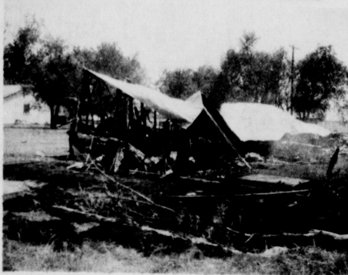
TOTAL LOSS: The trailer belonging to Mr. and Mrs. Glen Sherrell and family was a total loss as it was swept by fire Tuesday. The Wheeler fire department was called at noon. The Wheeler fire department was called to a fire Sunday night at 11:00 in Mobeetie; the concession stand at the ball diamond was destroyed. The cause of either fire is not known.
