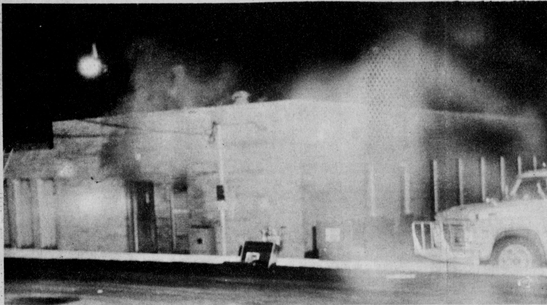
DENSE SMOKE—Smoke poured from the rear of the First National Bank in Bogata at the height of the early morning blaze, but prompt efforts of the
