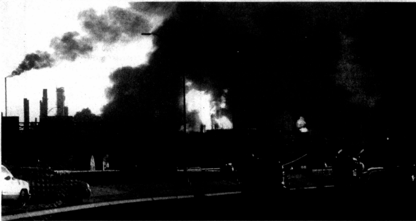
EARLY MORNING TRAFFIC was rocked by the explosion at the Alon (formerly Cosden) refinery in Big Spring early Monday morning. The explosion, which engulfed the plant in fire and smoke, injured five. Photo courtesy of Big Spring Herald .
