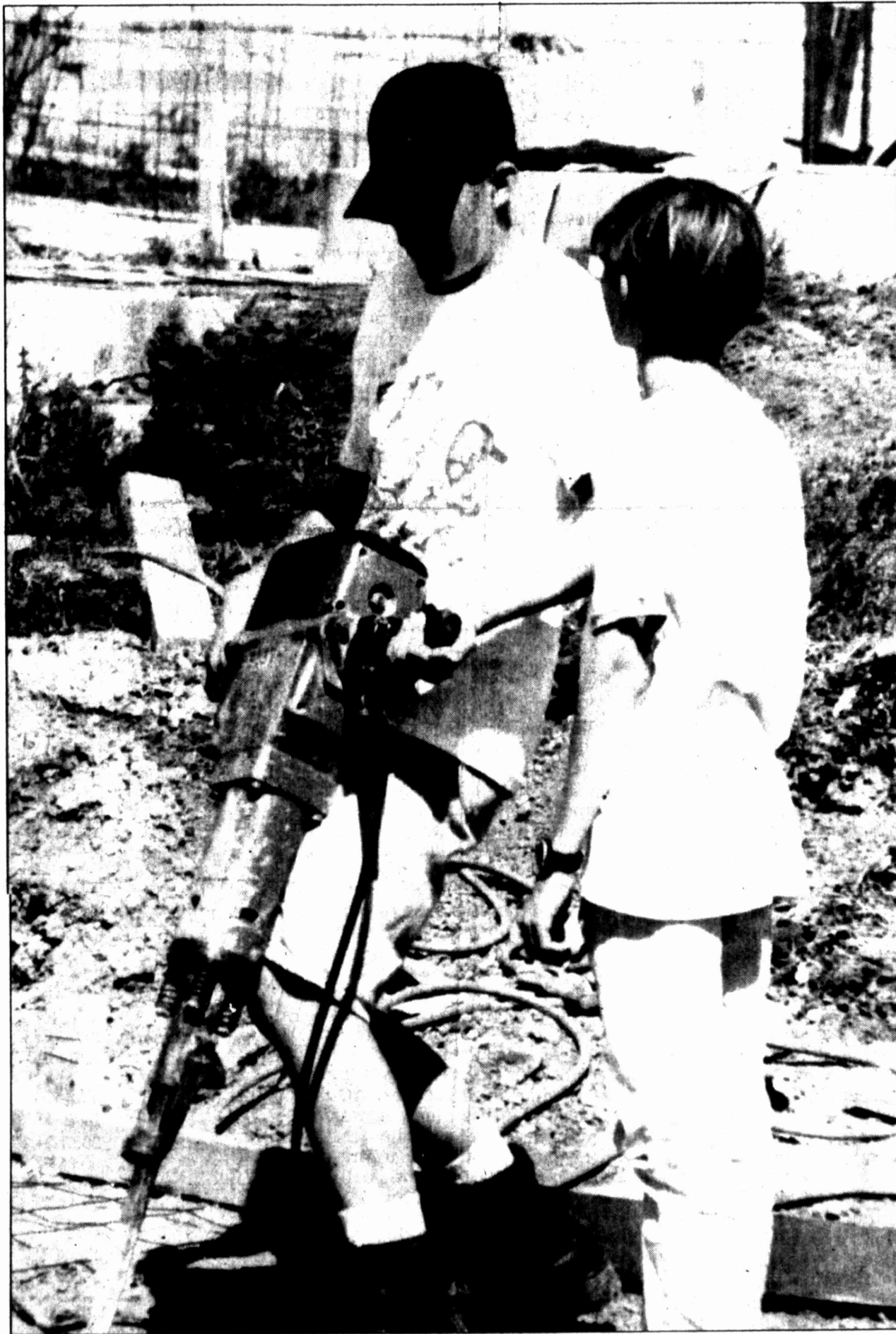
Marcus Fernandez operates a jackhammer, breaking out an old sidewalk while fellow scout Scott Downing looks on, as the two Scouts help on renovation of Big Spring's Boy Scout Hut. Fernandez, who spent the summer as a lifeguard and water safety instructor at the Buffalo Trail Council Scout Ranch, recently received his Eagle Scout certification.
