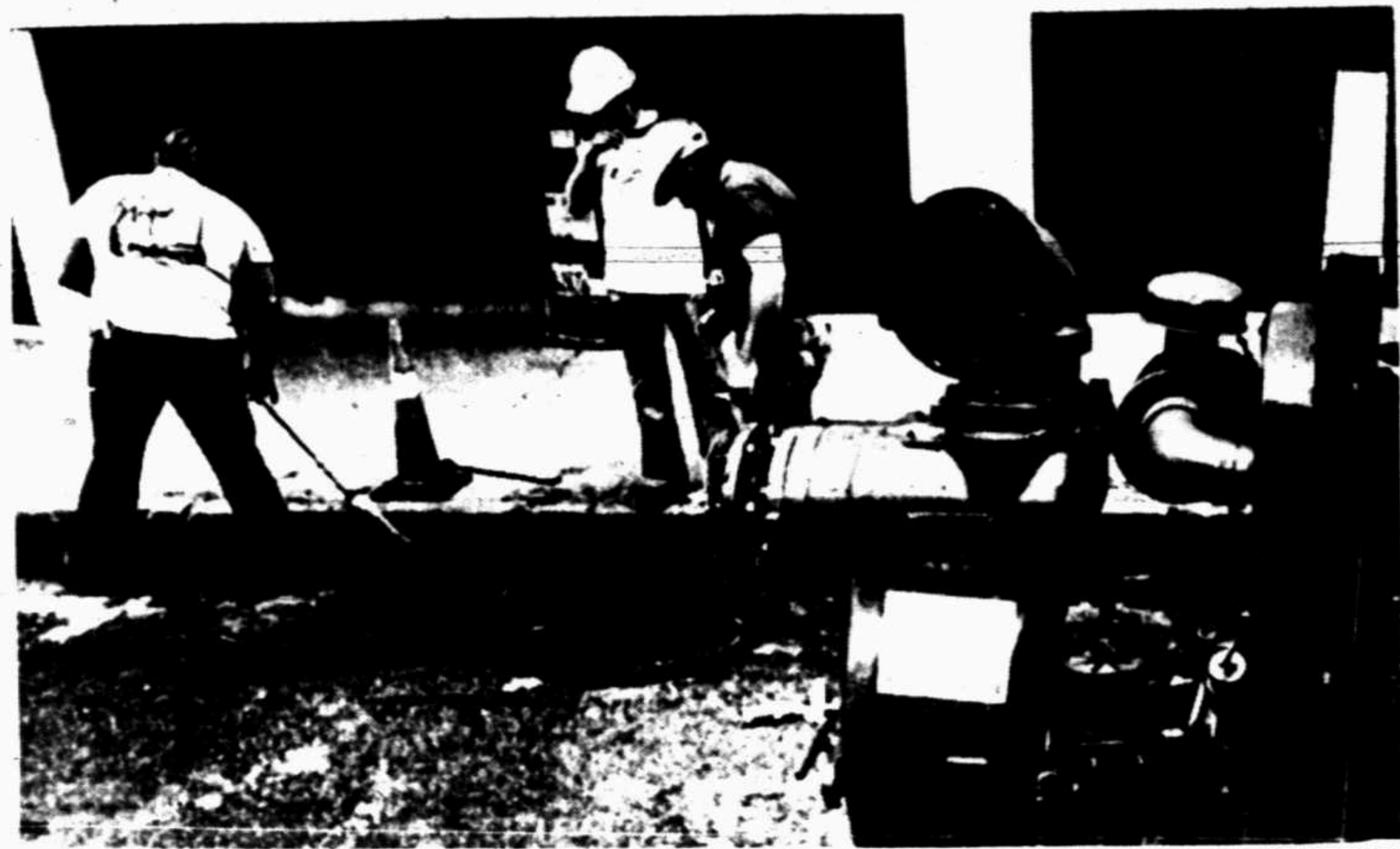
Workers inspect a flooded manhole next to a water pump outside the South Central Bell Building in New Orleans April 7, after an 11-inch rain. A flooded basement and failure of the $2 fuse crippled the city's long distance system for 10 hours and seared its link with a nuclear warning system.
