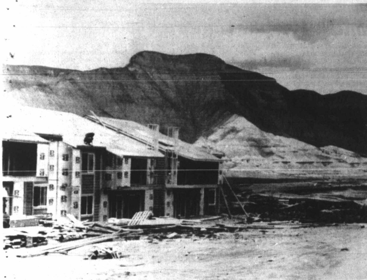
COLONY HOUSING. Carpenters continue finishing work on apartment complex in Battlement Mesa area of Colorado despite Exxon USA closing its huge Colony shale oil project. Builders are hopeful Union Oil shale
