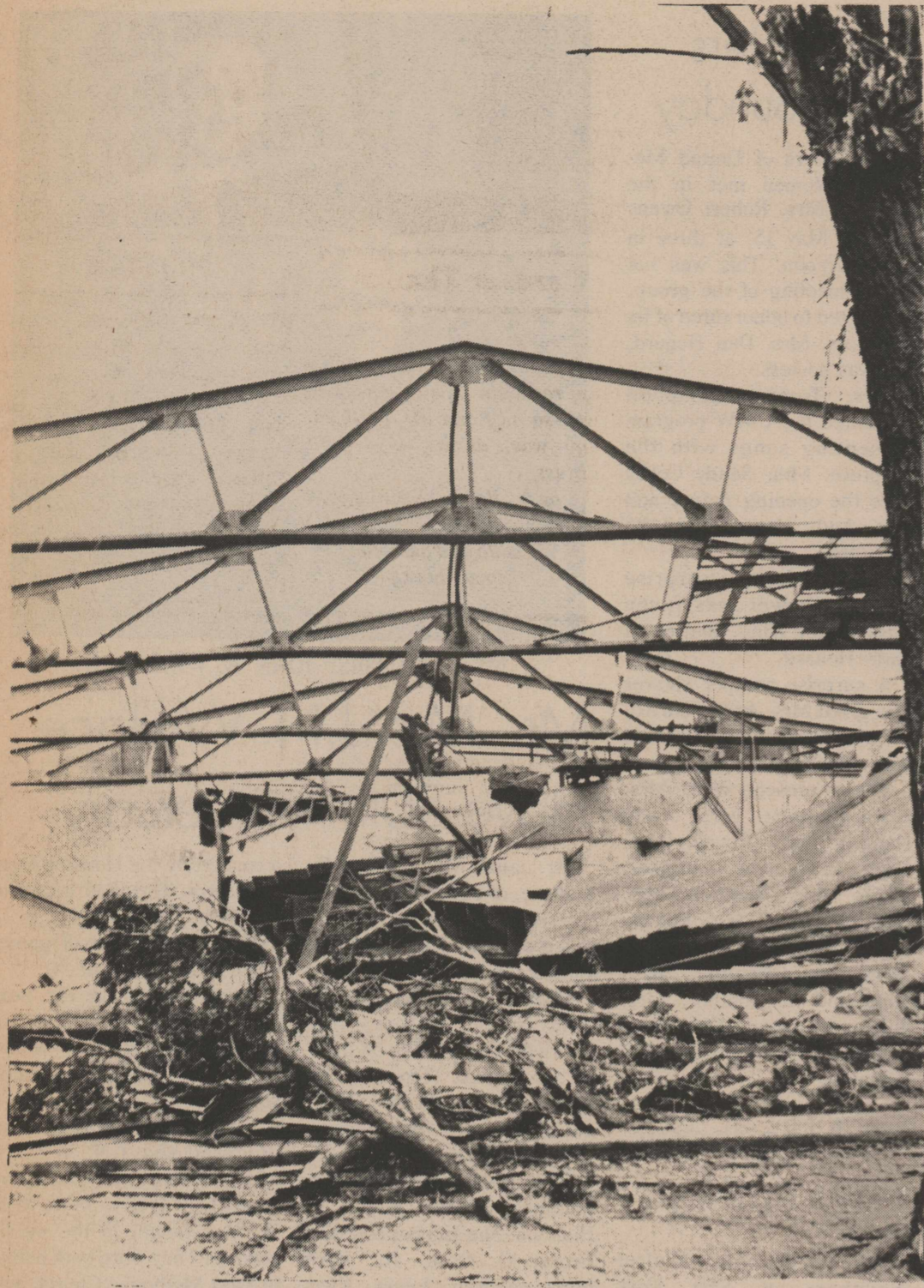
Rafters that echoed with hundreds of basketball games stand against the sky Monday, May 16 after a tornado ripped through the gymnasium of Quail School.
