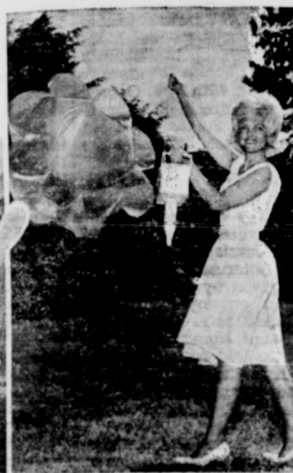
NORMA BURBRIDGE "test flies" new Bendix Friez Division upper-altitude weather instrument. Hundreds are used daily by the Air Force and the Weather Bureau, beaming information as they parachute to earth.
