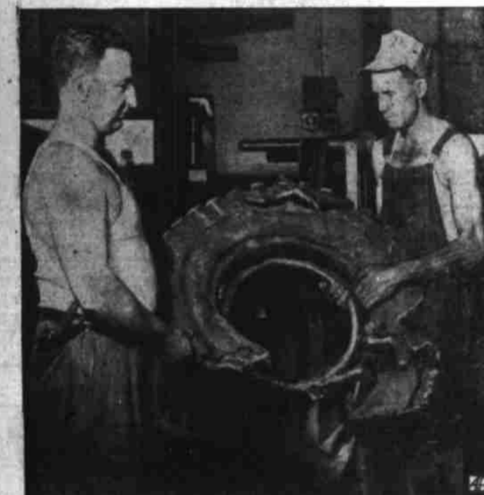
WOUNDED VETERAN. —Two tire builders in Good-year's Akron, O., plant look over remains of a 9.00 by 16 military tire, delivered to the Army in 1942, which was ruined by a Nazi land mine near Naples, Italy. Numerous carcasses like this were brought back to tire plants to show workers the urgent need for replacements on the war fronts.
