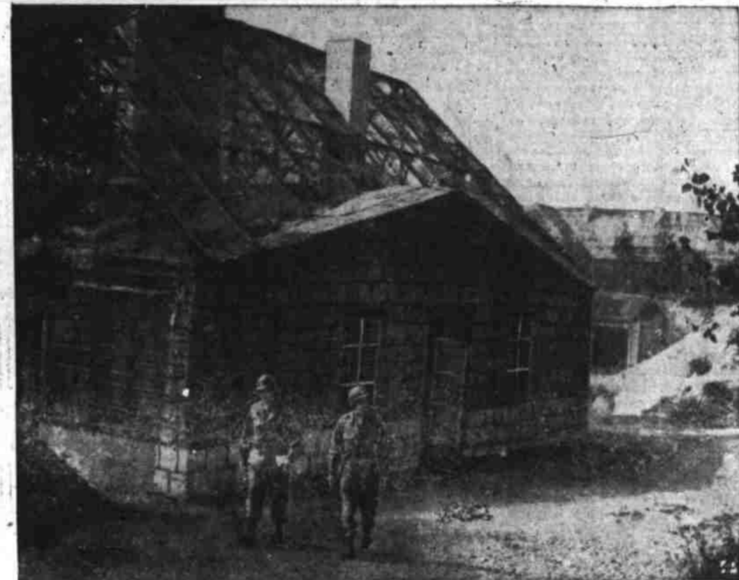
NAZIS' FAKE HOUSE. —Maj. Stanley Bach, Lexington, Ky., and Maj. James Hanley, Providence, R. I., inspect a "stone house" of plywood and netting built by Nazi camoufleurs in France.
