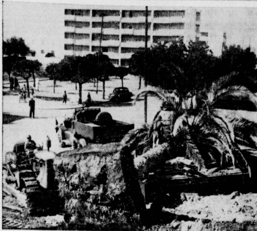
FOR A BETTER VIEW—Laborers and heavy equipment operators are working to make the quarters of the French air force officers more attractive in Rabat, Morocco. Palm trees were transplanted in order to give the men and their families something nice to see.
