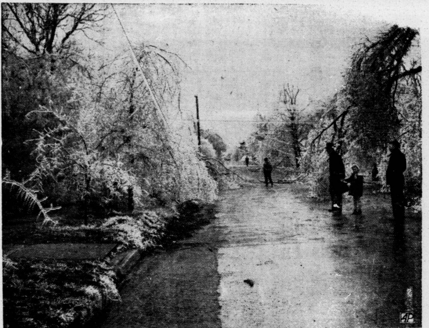
DENISON ICED IN —An ice storm which snapped communications lines and shattered trees over a wide section of North Texas left this street scene at Denison. Power was off throughout the city. Damage was heavy. (AP Photo).
