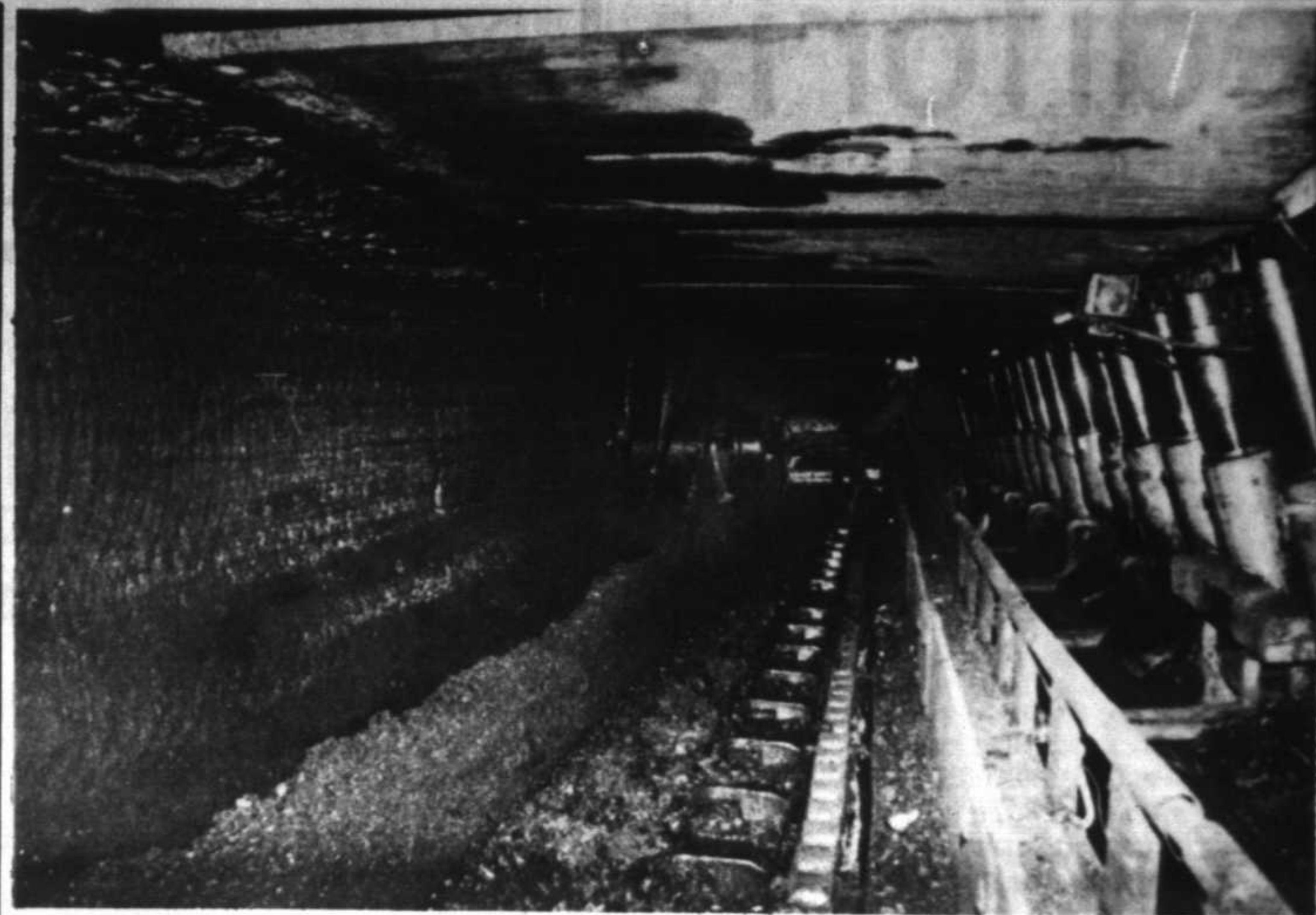
A miner watches as the shearer moves through a section of coal in a mine near Fairmont, W. Va. This method of shearing coal
