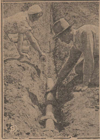
This sub-irrigated row in the garden of Rosa and Rudolph Smastria, East Barnard, Texas, furnished the family plenty of tomatoes for fall. Such irrigation systems are coming into use all over Texas. They are easy to install and lengthen the garden season.
