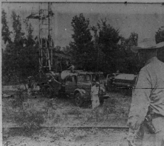
OIL WELL TESTED—Texas Ranger R. L. Badgett stands watch as a crew begins to test an oil well near Greggton for possible deviation. The Texas Railroad Commission is in the process of testing several wells in the rich East Texas fields. (AP Wirephoto)
