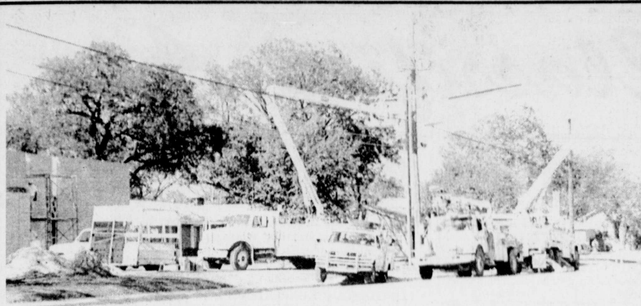
WTU CREWS work efficiently to install a transformer and electric lines to the new First Baptist Church Fellowship Hall. Ordinarily this job would have lasted a couple of days, but with a number of trucks and added manpower this job was completed in less than a day's time.
