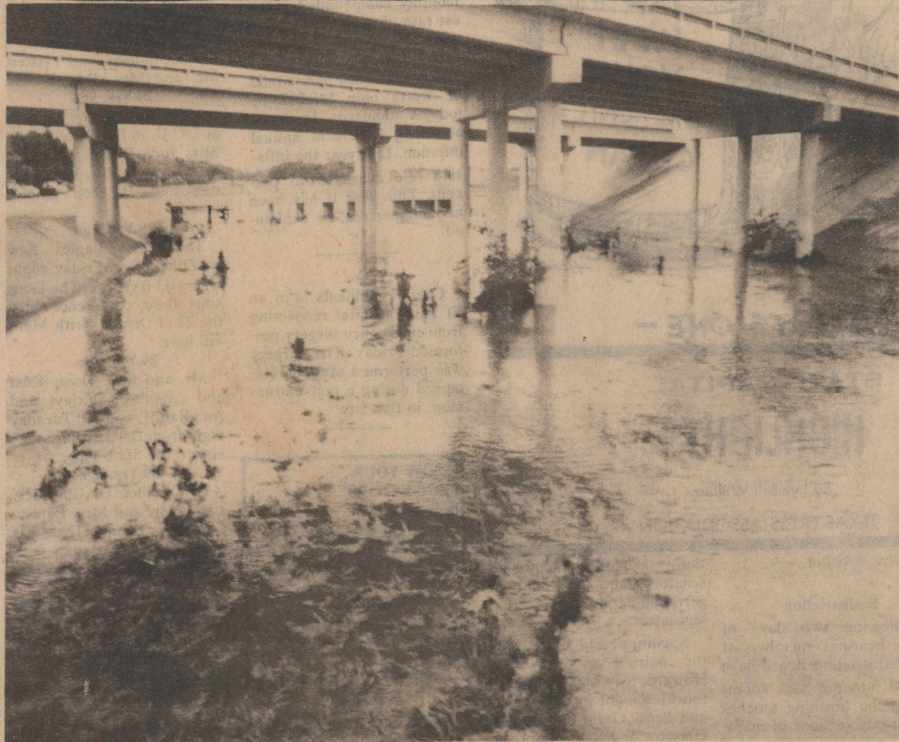
RAINS TURN DRAWS INTO RIVERS, and the only way to get across town in Ozona Monday morning was the 1-10 bridges over the interstate or the bridge across Johnson Draw. Over three inches of rain during the night Monday
