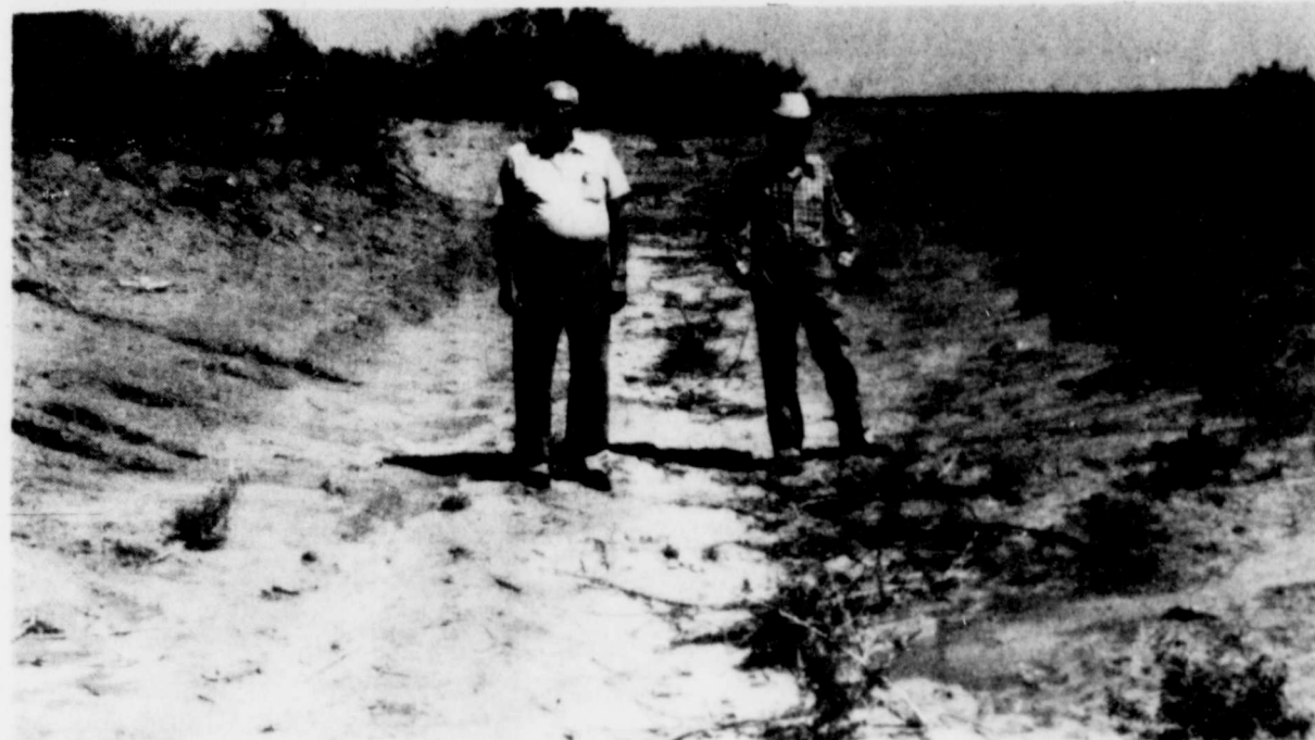
BILL GREENE, left, and Van Mills are standing in the channel of a diversion constructed by Mr. Greene.
