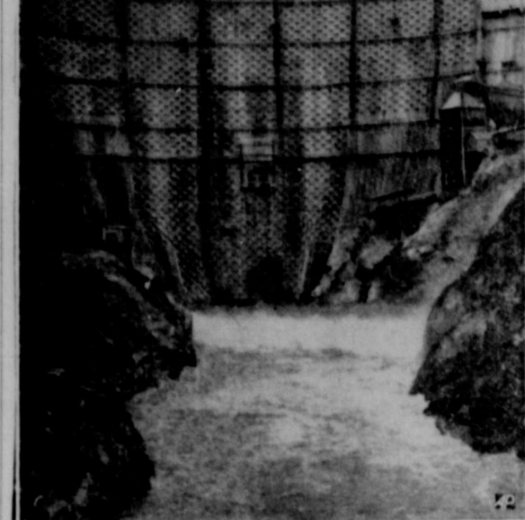
SEATTLE 'WAFFLE'—Seattle has a $28,000,000 "waffle" standing on edge in the Skagit river, 130 miles north of the city. It is a giant Ross dam, towering 405 feet above the floor of the Skagit gorge. The above view shows the dam from the downstream angle. The indentations in the dam are five feet square and two feet thick. The waffle indentations were left because the engineers plan some day to add to the dam, and will pour new cement into the holes in this one.
