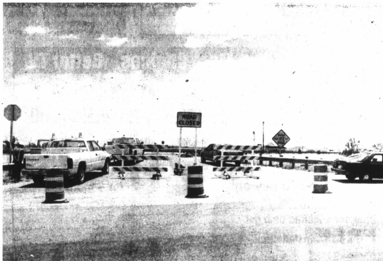
BRIDGE CLOSED -- Overpasses at both the north and south edges of town are closed for construction for the next three months. Shown here is the cemetery overpass on the southern edge of Tahoka, and the FM400 overpass on the north edge of town is also closed. (LCN PHOTO)
