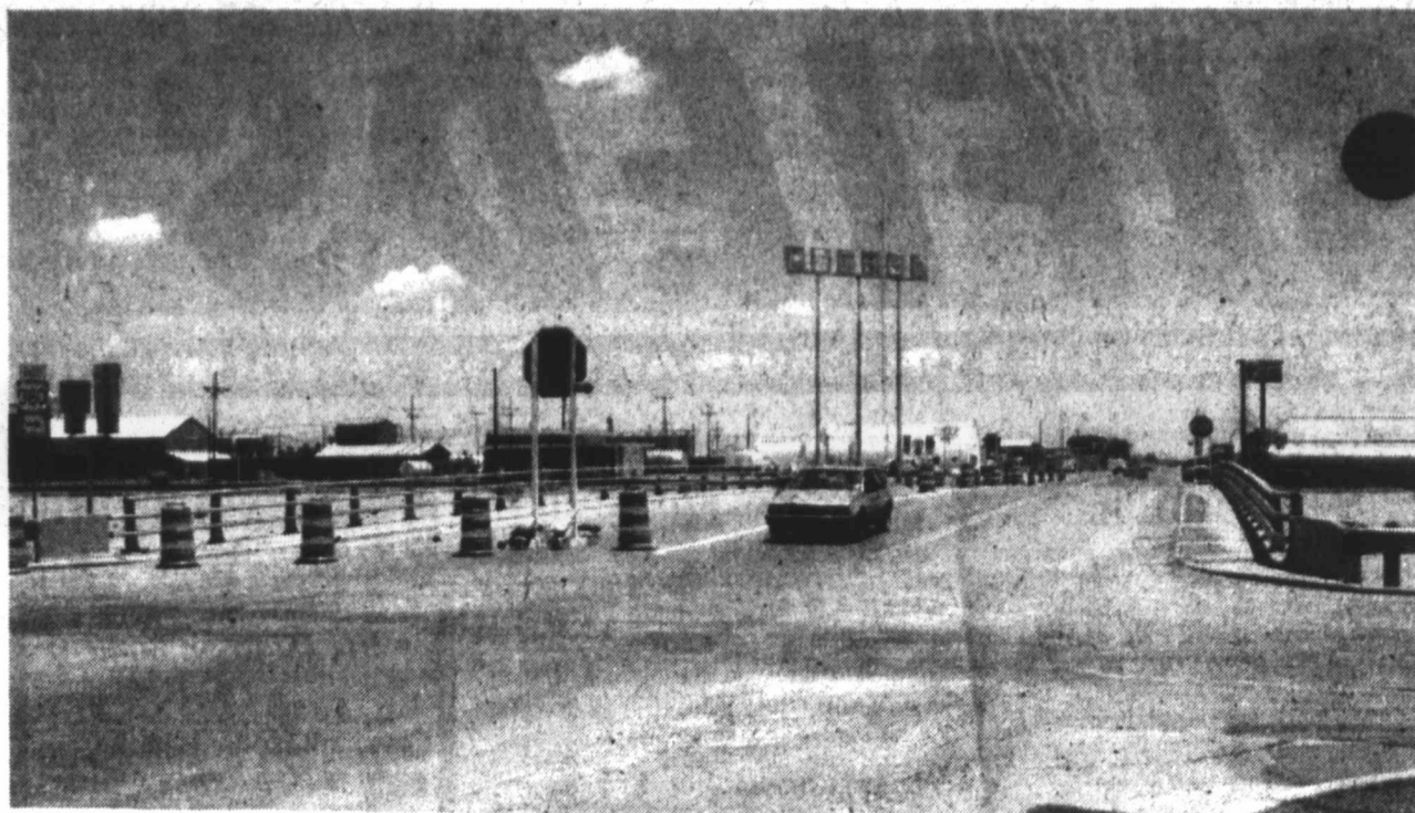
BRIDGE DIVIDED - The north half of the Hwy 380 overpass in Tahoka is blocked from drivers during construction, with traffic diverted onto the southern half of the bridge for both east and westbound traffic. Bridgework is expected to be under construction for the next three months. (LCN PHOTO)
