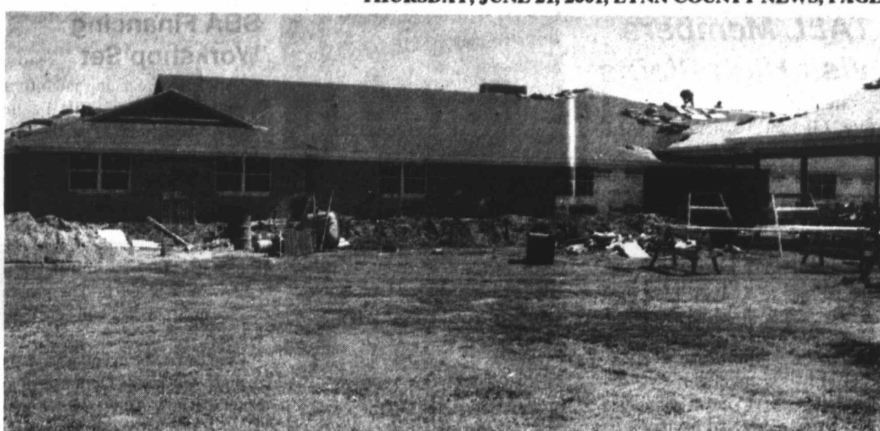
BRICKING IT UP - Exterior work is giving the Lynnwood Assisted Living Center a more finished look this week, as construction continues on the project. Located just north of Lynn County Hospital District in Tahoka, the center will offer 20 apartments for older citizens who need an alternative between living alone at home or going into a nursing home. The center is expected to open this fall, and will be operated under the auspices of Lynn County Hospital District. (LCN PHOTO)
