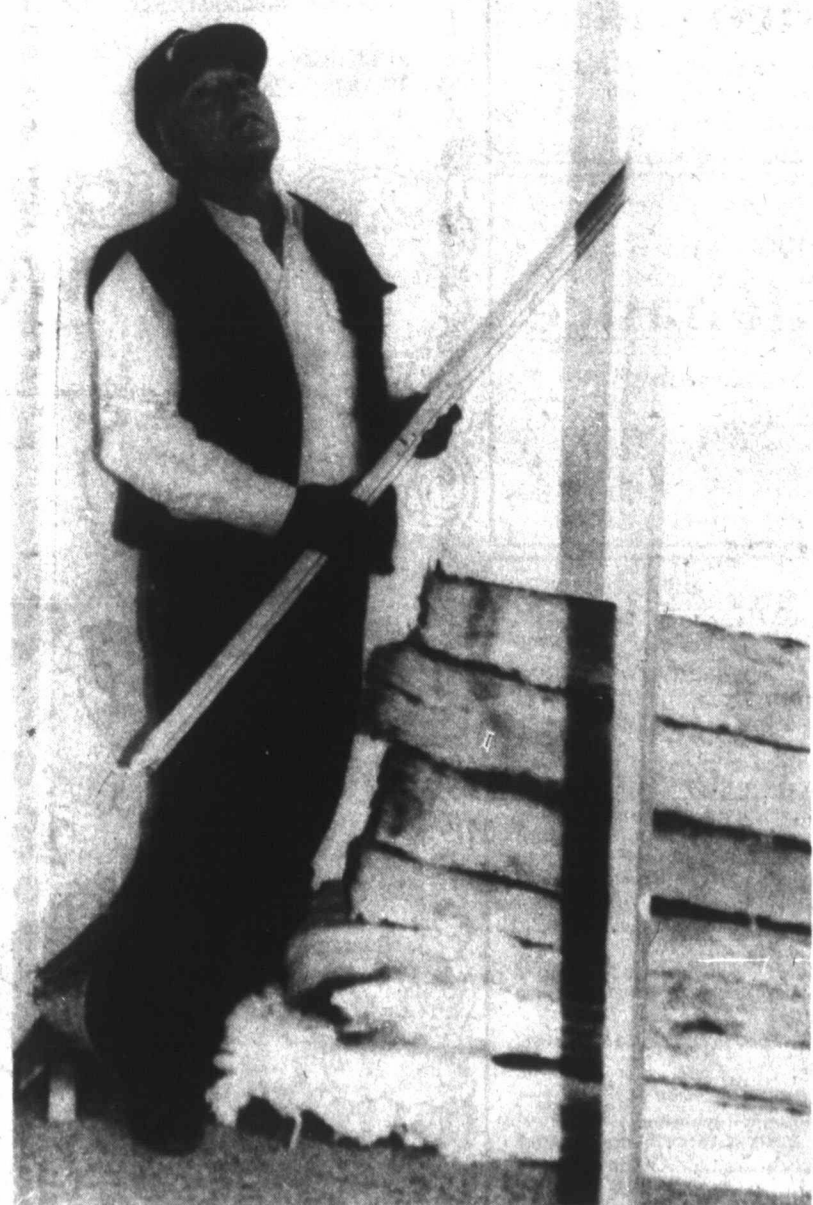
AUXILIARY SHOP BEING ENLARGED: The Pink Ladies Auxiliary Shop at the Mitchell County Hospital is being expanded by employees of the hospital. Cecil Contreras is shown doing some of the work Friday.
