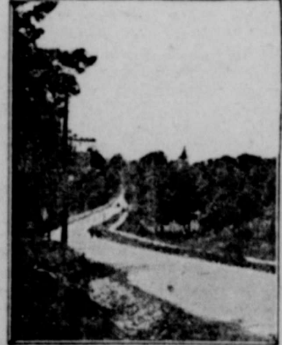
A Completed 20-Foot Concrete Road.
