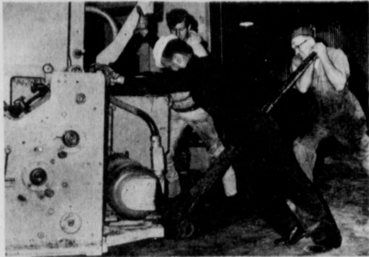
Folder unit manhandled into new building.
