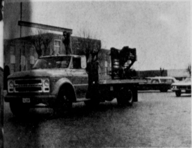
First of four units heads for new location.
