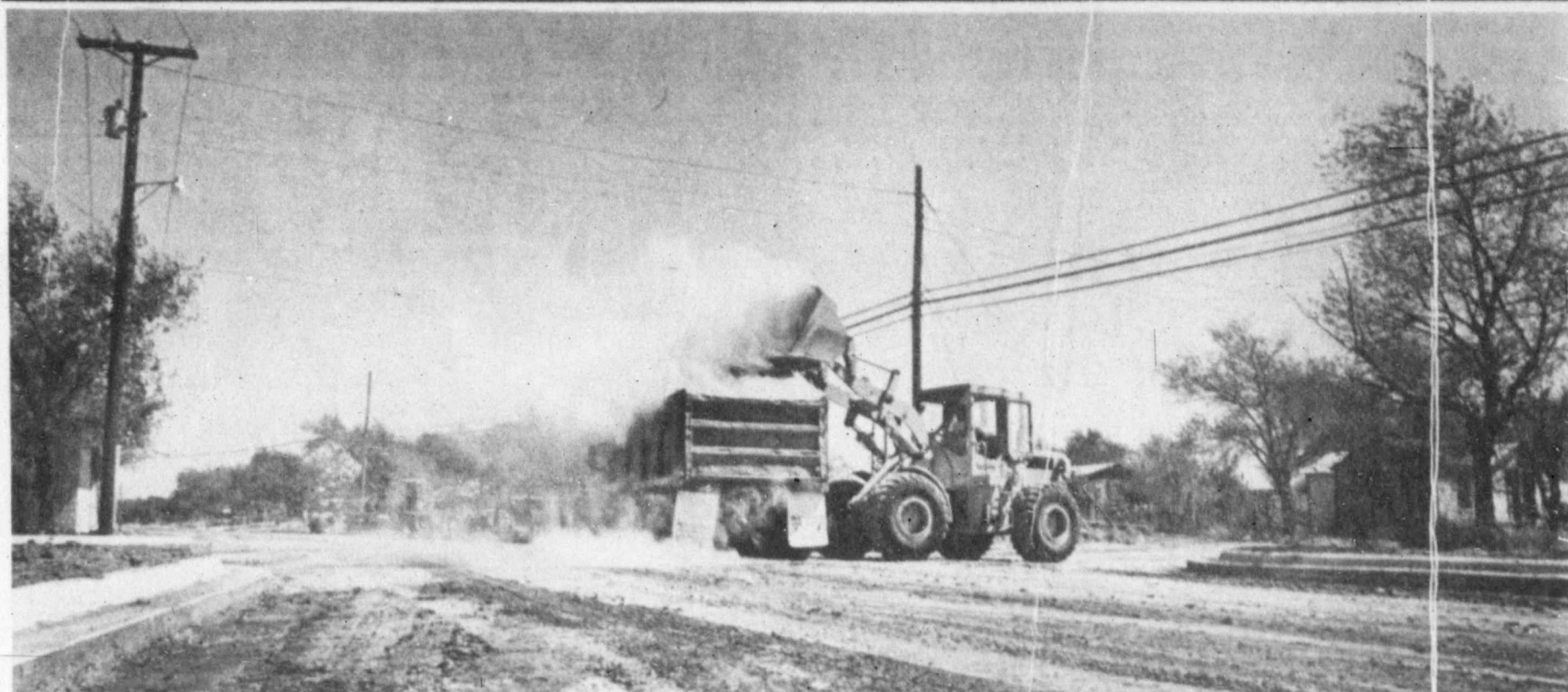
City crews work on a paving project on New York Avenue funded by a Community Development Grant. Although it is doubtful there will be more Community Development money, city officials said Tuesday there were other means to complete paving projects in east Midland. (Staff Photo by Jim Steinberg)
