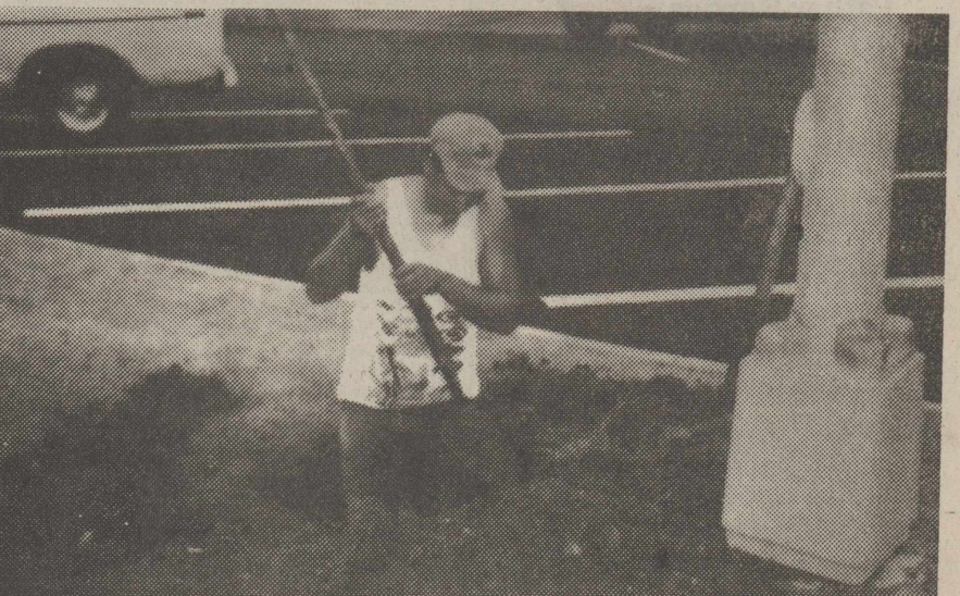
DIGGING A HOLD: Gilbert Ramirez, Rotan City employee, was busy digging holes in the center median to install new sprinklers last week. A total of approximately 15 sprinkler heads will be installed in the near future.
